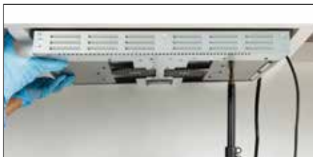
Attach the system to the porcelain slab using a prop while keeping a space of 5 cm to 10 cm on both sides for proper airflow.
